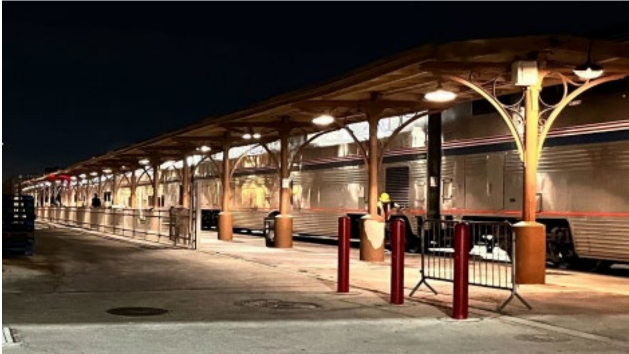
Figure 11: The current platform, visible are the low floor requiring steps and the end of the awning.
